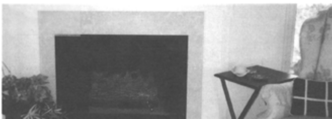
Figure 1. Ghosting stains have been seen on interior and exterior wall surfaces; on carpet surfaces at wall-to-floor connections or door undercuts; on ceilings; on furniture, around wall and floor coverings, and numerous other places (1). For a stain to appear, two factors must be present. There must be a source of particulate matter, like the carbon soot from candles or gas log fireplaces (2) and there must be a driving force, like gravity, electric attraction, or a forced air unit (3) to push the particulate against a surface.
